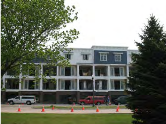
Hancock, Pentwater New Infill Condominiums
