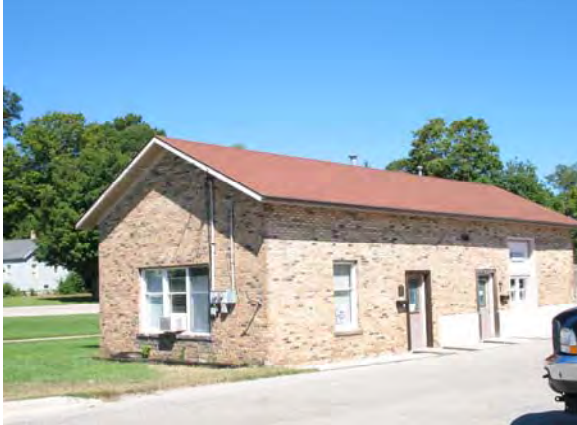
Fifth Street, Shelby Chesapeake & Ohio Railroad Building
