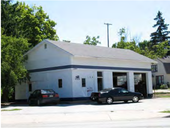
Sixth Street, Shelby Former Texaco Gas Station
