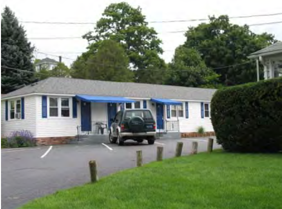
710 W. Ludington Avenue, Ludington Lighthouse Motel
