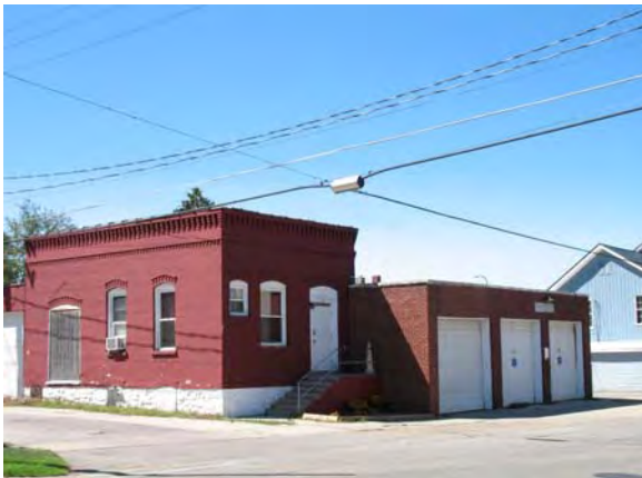
25 Third, Shelby Fire Station
