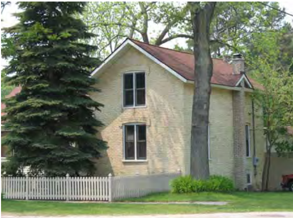
U.S. 31 Business Route, Pentwater Pentwater Brick Residence
