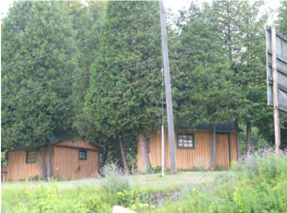
1743 Pere Marquette Highway, Ludington Cedar Ridge Cabins
