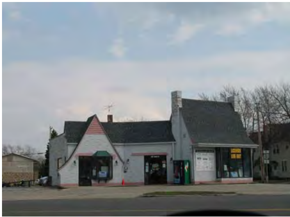
1127 Main, Saint Joseph Gas station
