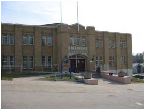
472 Cass Street, Benton Harbor Bobo Brazil Community Center
