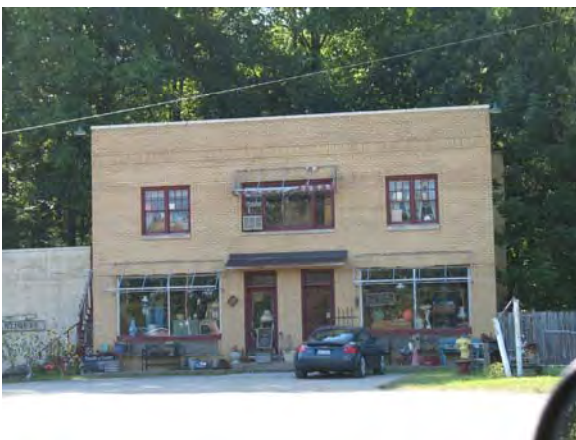
Red Arrow Highway @ Holloway Road, Sawyer
