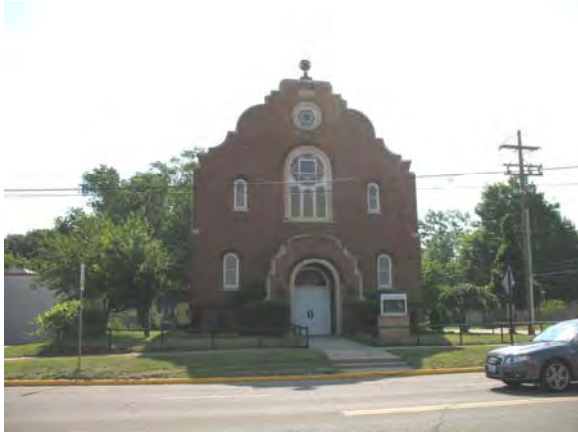
249 Broadway, South Haven First Hebrew Congregation of South Haven
