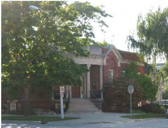
500 Main Street, Saint Joseph Allegretti Architects Office Building
