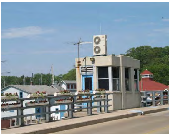
Dyckman Avenue over the Black River, South Haven Bascule Bridge
