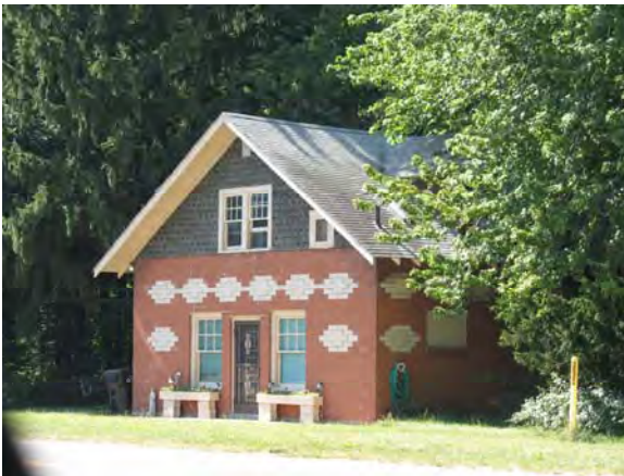
Red Arrow Highway, Harbert
