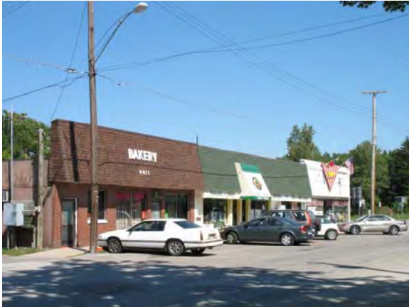
9805 Union Pier Road, Union Pier G & K Party Store
