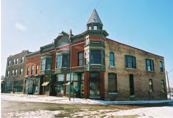
Water Street, Benton Harbor Hinckley Block
