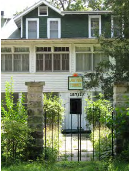
15711 Lakeshore, Union Pier Lakeview Terrace
